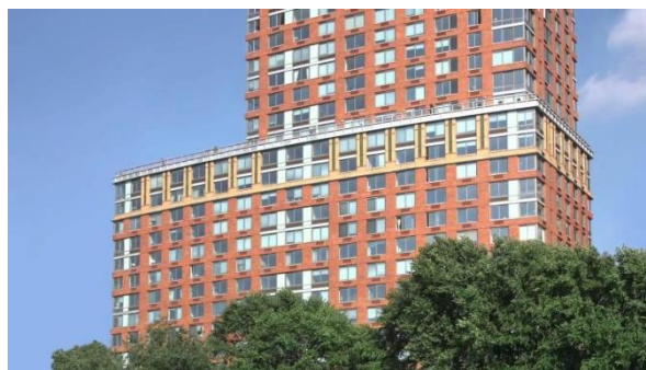
3-rasm. "Twenty River Terrace" binosi, bino fasadiga o'rnatilgan quyosh panellaridan foydalanish
